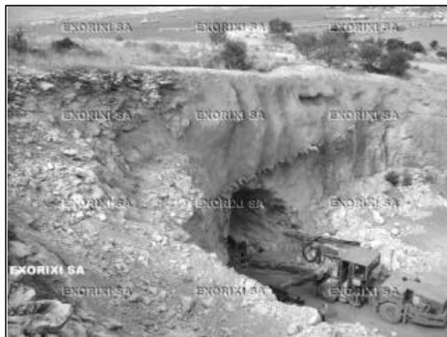
This short in length tunnel is an underground passage on the New Peripheral Motorway of Aegaleo. This tunnel has been designed because of the findings that are on the surface, just 7m over the excavation roof: part – remains of an ancient road (“Sacred Road” is more than 2.300 years old), a distributing natural gas main and a network of distributing fuel pipelines (an oil refinery and military facilities of fuel storing are located close to the project).
